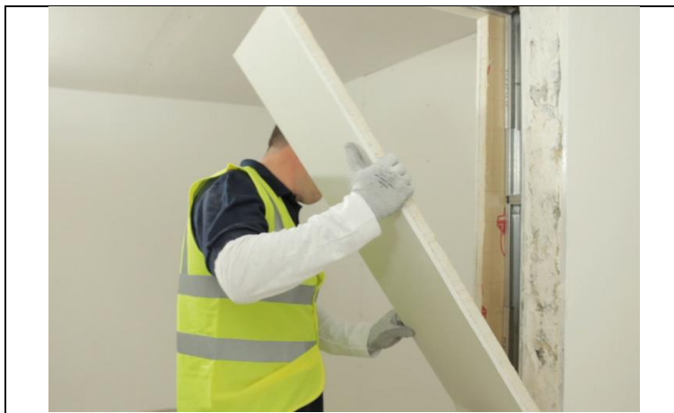
Figure 4 Window reveal installation
