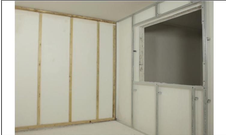
*Figure 4 Window reveal installation*
